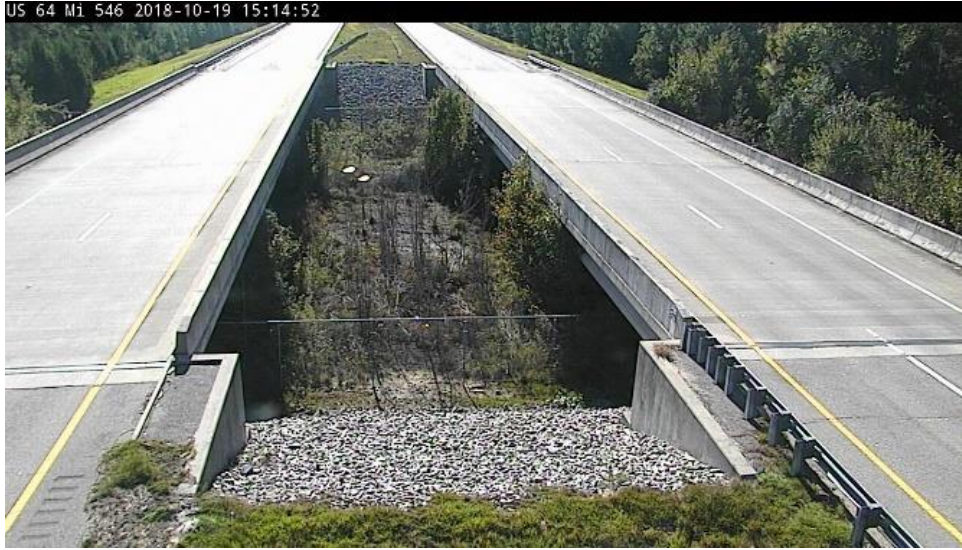
Figure 13. Wildlife underpass on US 64 in Washington County.
