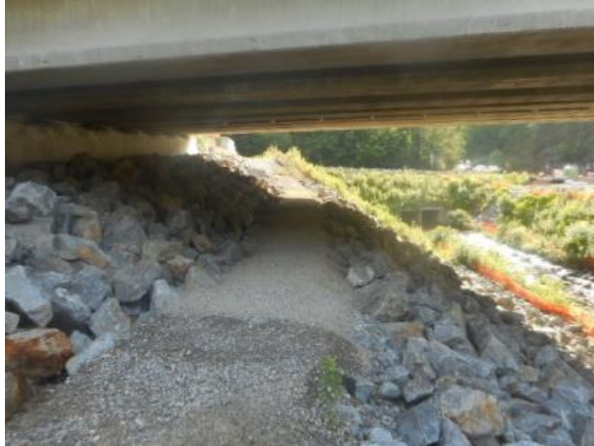
Figure 9. Wildlife pathway or "bench" as-built from Figure 8.
