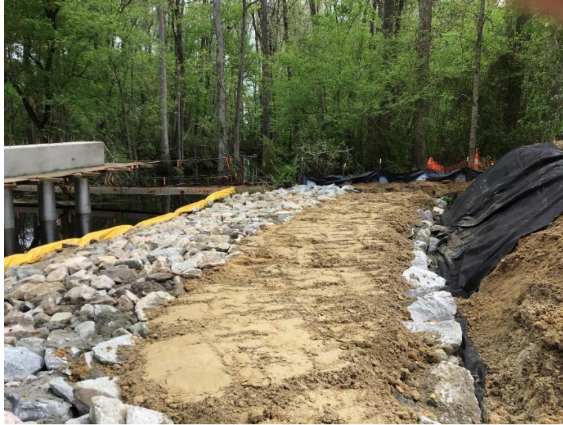
Figure 11. Construction of bench over embedded rip rap (Edgecombe County, # 320113, Otter Creek).
