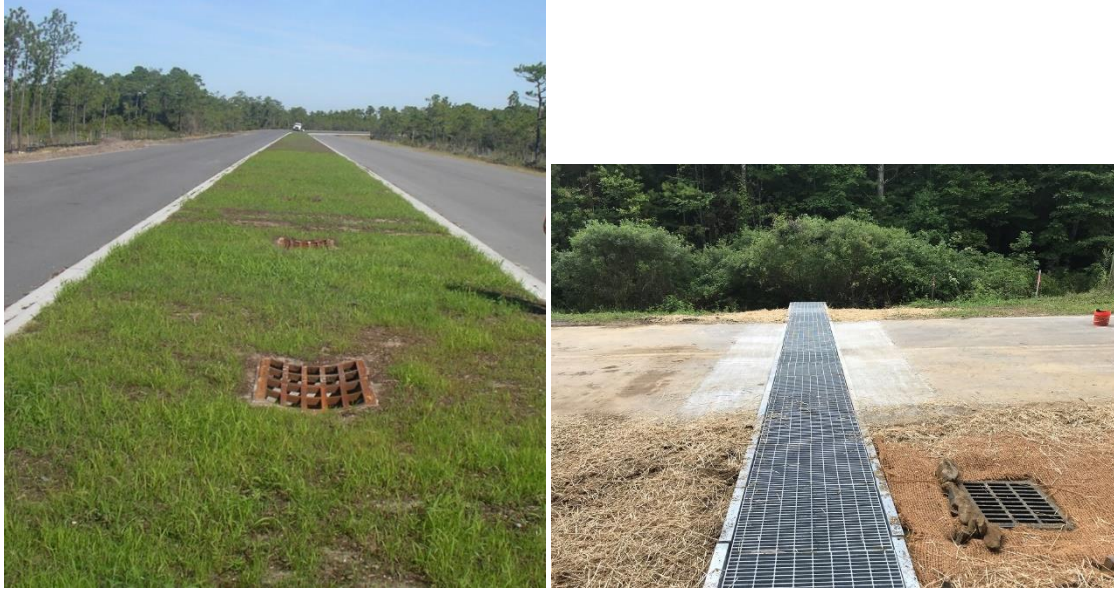
Figures 18 and 19. Grate in median of wildlife culvert, EF Middleton Blvd Brunswick County (left) and open grate crossing Ash County.
