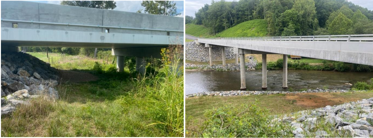
Figures 6 and 7. Unarmored floodplains under bridge in Iredell County (left, #480212, Patterson Creek) and large bridge in Stokes County (right, #840008, Dan River)
