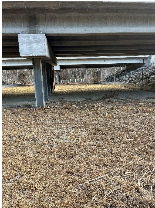
Figure 14. Wildlife underpass on US 17 in Jones County for connecting habitat for range of species.
