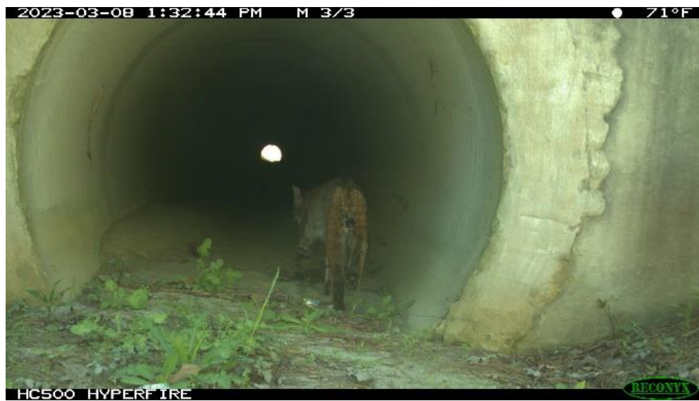
Figure 17. Daylight visible through culvert, US 17 Wildlife Crossing Jones County.
